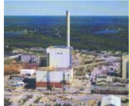
The Alholmens Kraft biofuelled power plant in Pietarsaari, Finland is one of the largest in the world. The plant is a CHP facility producing electricity for the owners as well as steam that is used by a nearby UPM mill and by the local municipality for district heating. The plant is designed to use 150,000 to 200,000 cubic meters of loose or bundled logging residue annually. Photo: TEKES brochure 2002
