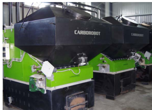
High-efficiency Heat Only Boilers
