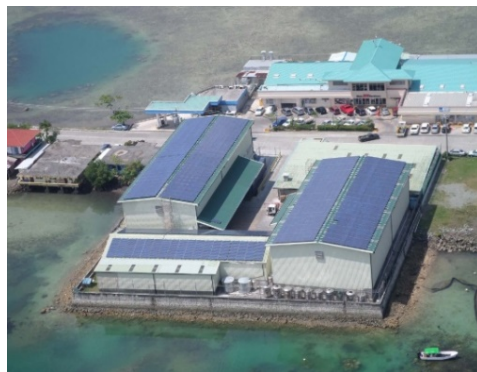
Solar Power Plants
